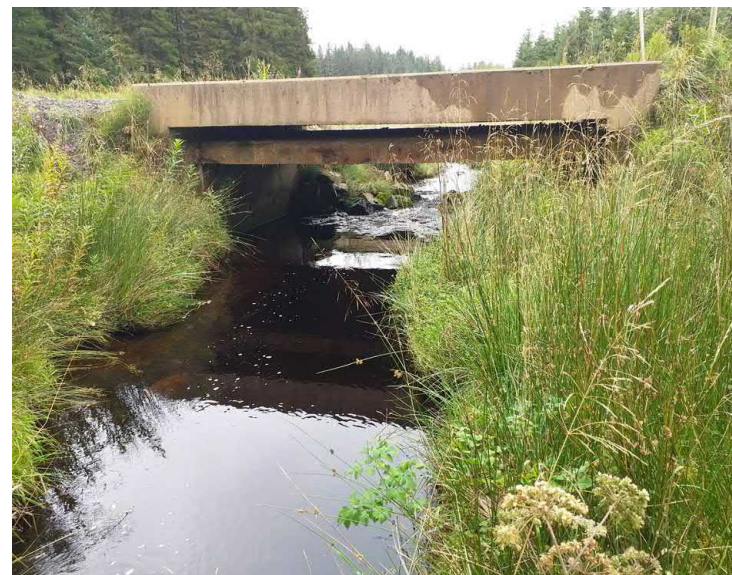
Looking upstream from NGR 300825, 596580
